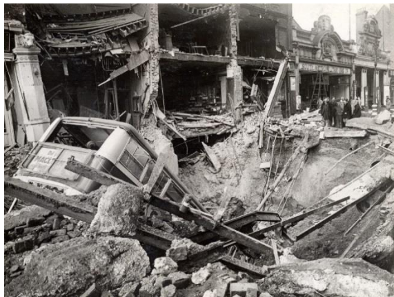
AFTERMATH: 88 bus sits amid the wreckage on Balham High Road
